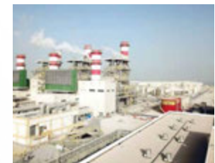
UMM AL HOUL POWER PLANT (Qatar)
