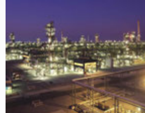
GASCO HABSHAN PROJECT (United Arab Emirates)
