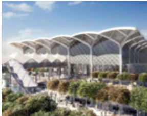
HARAMAIN HIGH SPEED RAILWAY MAKKAH STATION (Saudi Arabia)
