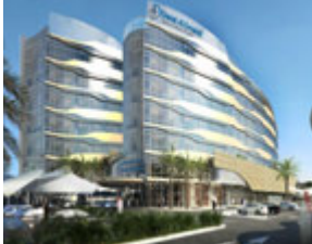
DANAT AL EMARAT HOSPITAL (United Arab Emirates)
