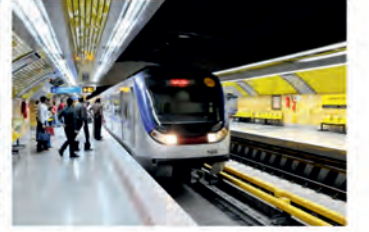
Tehran & Shiraz Subway Stations Tehran & Shiraz / Iran
