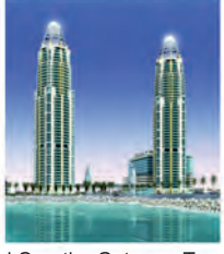
Abraj Quartier Gateway Towers Doha / Qatar
